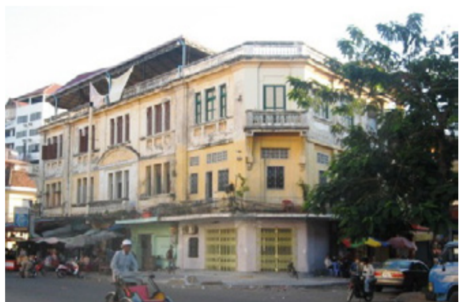
The Grand Hotel. The back of the building, current state
