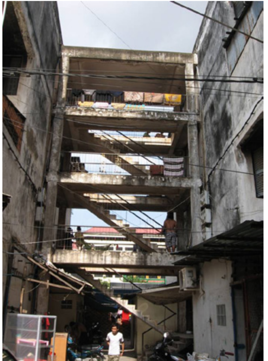
A stairway of the Building
