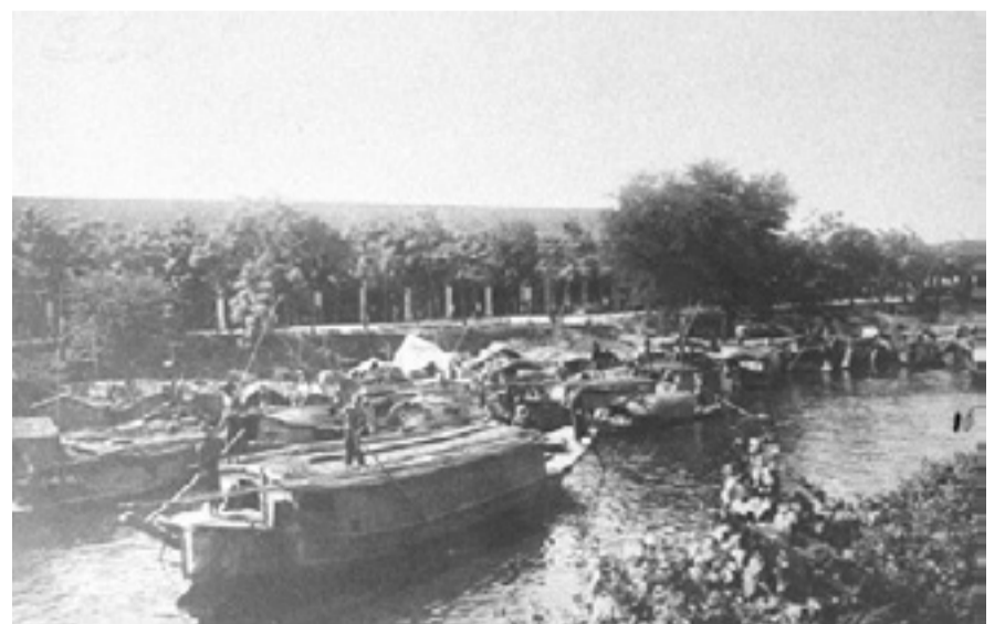
The western part of the canal
