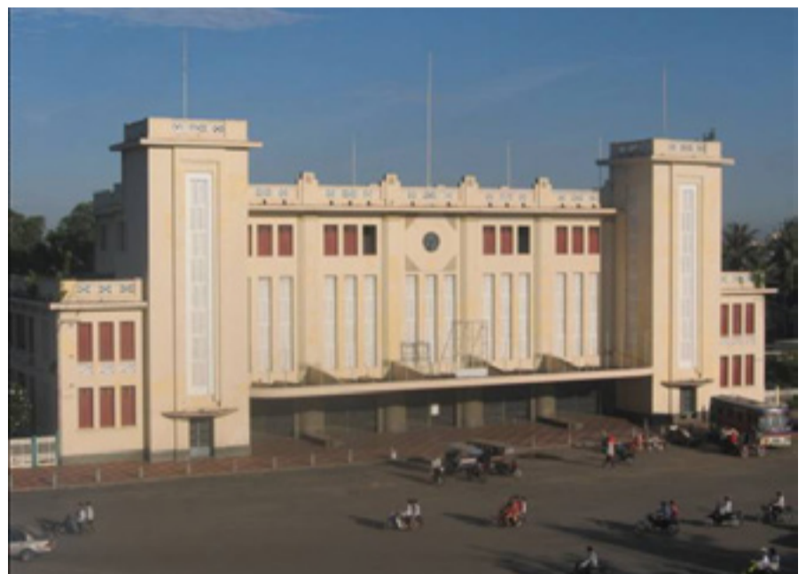
The railway station, current state
