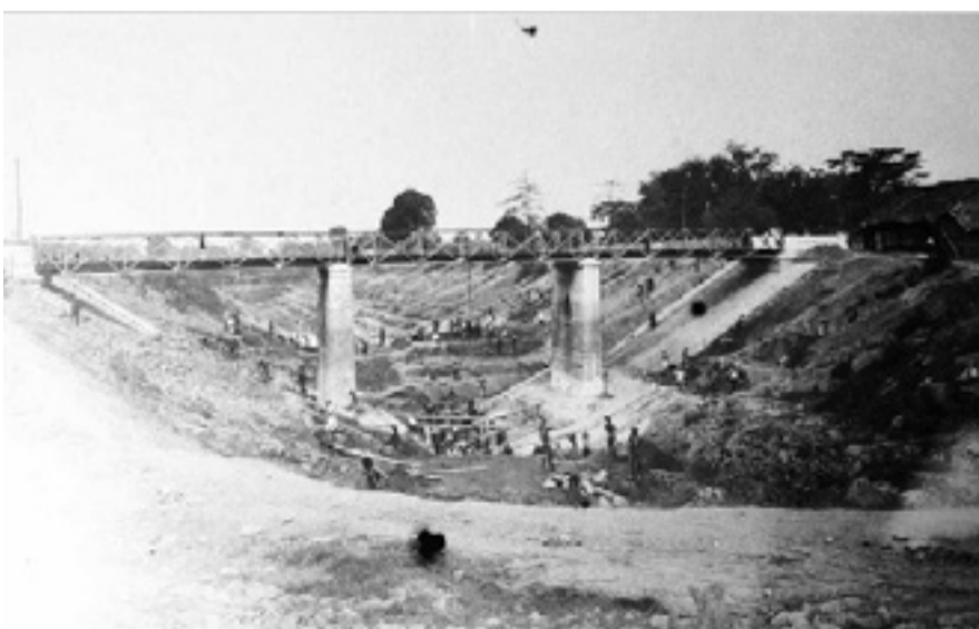
Ohier bridge. Currently a section of Street 13
