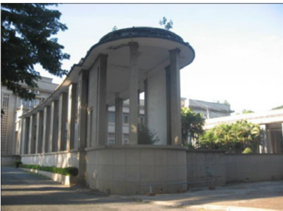
The new one which replaced it in 1934, today the Center for Development of Cambodia
